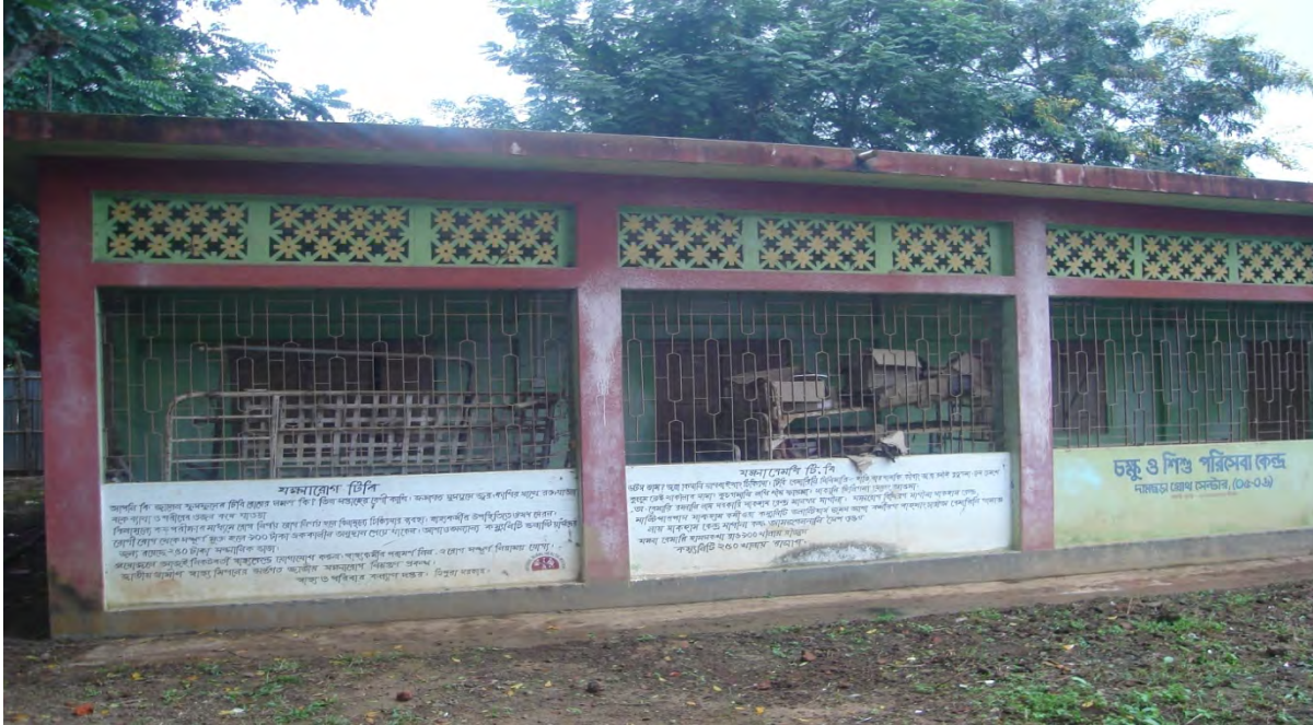
(At Damcharra PHC: Large part of building lying idle)
